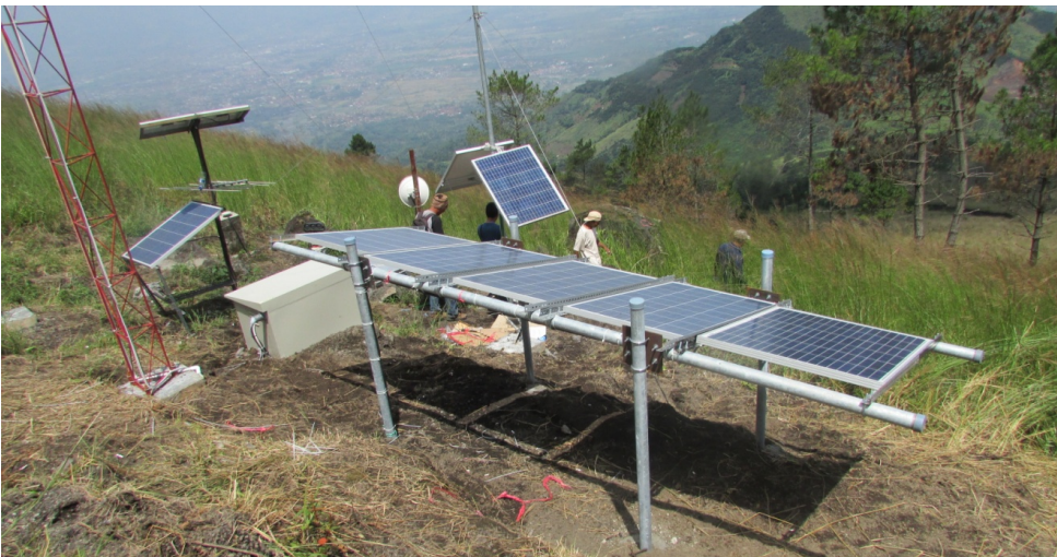
Adding Solar cell at Sodong Station
